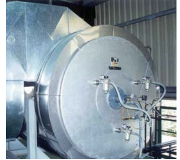
Thermal oxidation chamber
