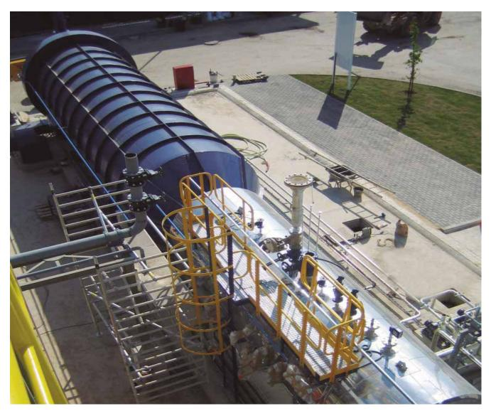
Recuperative thermal oxidation is a technology that carries out the destruction of volatile organic compounds in an oxidation chamber, providing adequate conditions of temperature, residence time and turbulence of the mixture.
